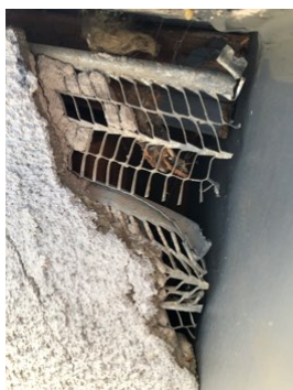
Exposed eave stucco lath with no backing
