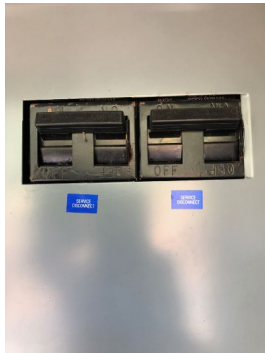
200 amp X 2 main breaker detail
