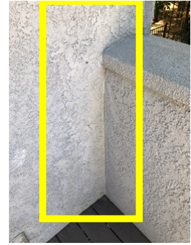
Stucco patch on master deck area
