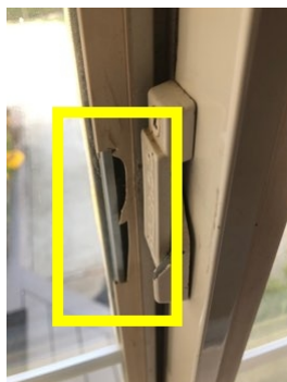
Damaged bedroom 4 exterior door
