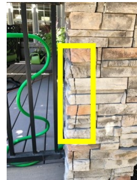
Deck railing stone column cracking
