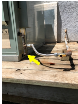
Gas line with sediment trap
