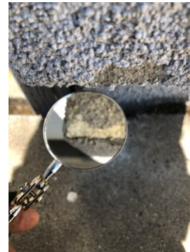
Exposed bottom foam on front trim
