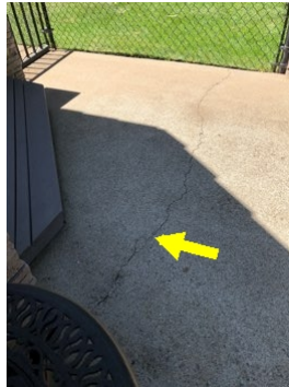
Right side patio cracking
