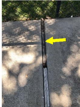
Wood decay on right patio expansion joint
