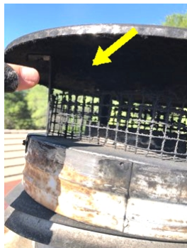
Large gap in spark arrestor
