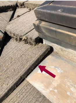
Skylight flashing under tile
