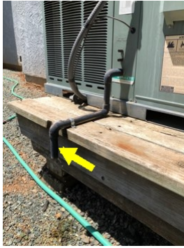
Missing trap on condensate drain line
