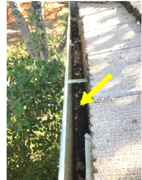
Gutter clogged with organic material
