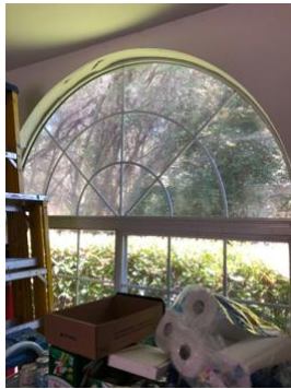
Possible failed seal
