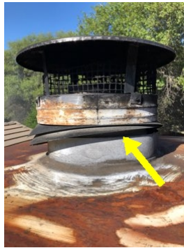
Loose chimney flue collar
