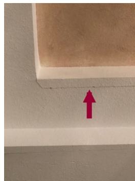
Dining room ceiling crack
