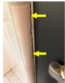
Deficient back wall seal
