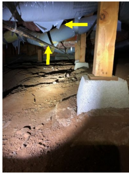
Torn duct pipe vapor barrier
