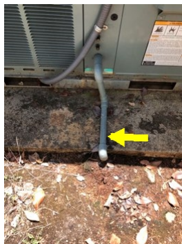
Missing trap on condensate drain line
