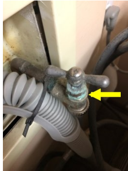
Corrosion on washer water valve
