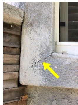
Window trim cracking
