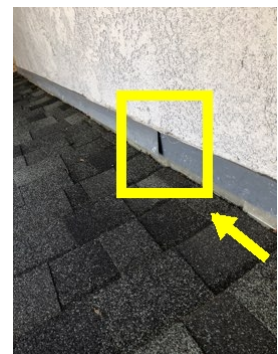
Wrong overlap on stucco sidewall flashing
