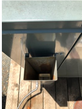
Missing exterior vent screen
