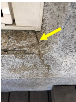
Rear right window trim cracking
