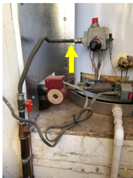
Gas line without sediment trap
