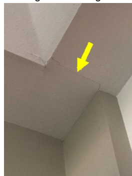
Living room ceiling crack
