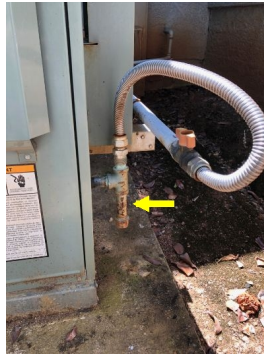
Gas line with sediment trap
