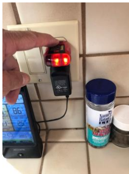
Deficient counter GFCI outlet
