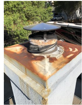
Rusted metal chimney crown
