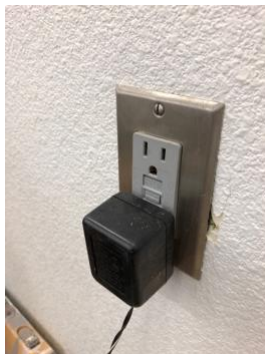
Right GFCI protected outlet
