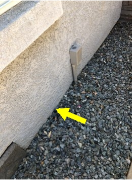
Weep screed covered on right side
