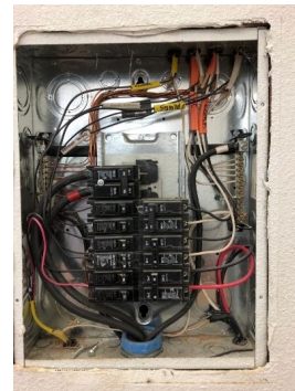
Detached garage sub panel detail
