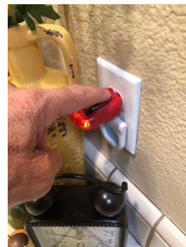
Deficient bath 3 GFCI outlet
