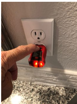
No half bath outlet GFCI protection
