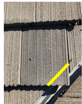
New tile not cut for valley flashing
