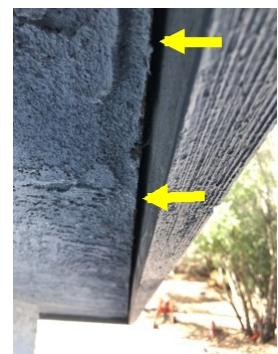
Stucco separation from barge rafter
