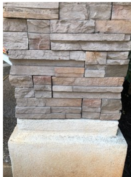
Drain plane not evident on columns
