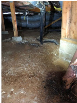
Damp crawlspace soil
