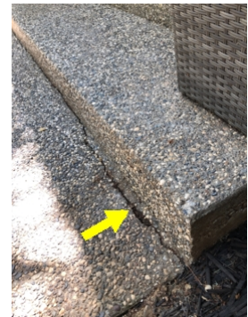
Concrete entry stair base cracking
