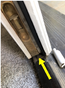
Living room inactive door would not open
