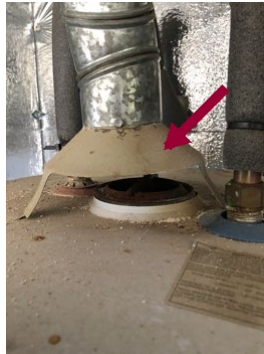
Misaligned vent pipe
