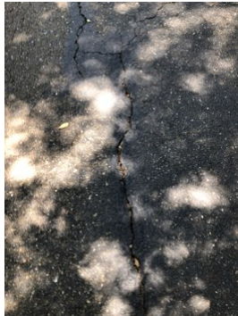
Asphalt driveway cracking
