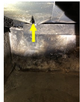
Broken firebox brick
