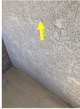
Rear stucco cracking
