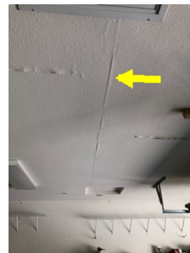
Lifting seam tape
