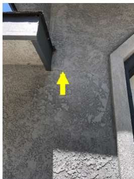
Front stucco crack
