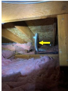
Interior moisture exhaust pipe detail
