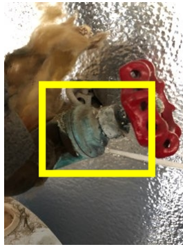
Corroded water shut-off valve
