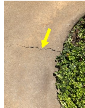
Rear patio cracking
