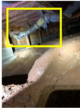
Torn duct pipe vapor barrier
