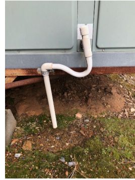
Example of proper condensate trap
