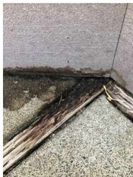
Right side landing moisture damage
