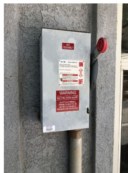
Main disconnect possibly for generator use
