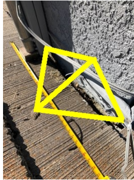
Missing cricket to divert water
