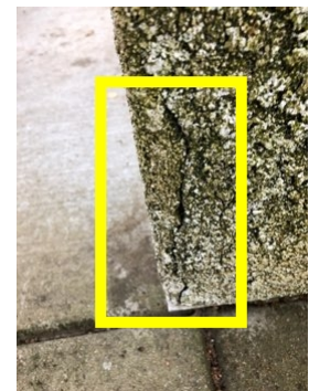
Rear stucco corner crack
