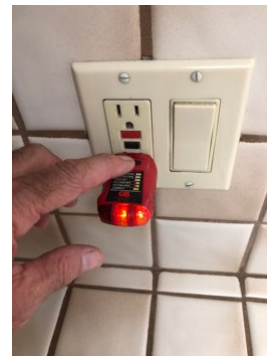
Deficient counter GFCI outlet
