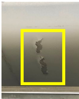
Peeling ceiling paint
