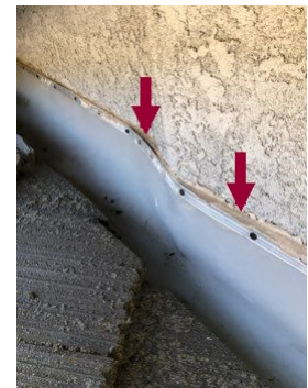
Questionable sidewall flashing
