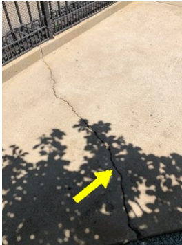
Right side patio cracking
