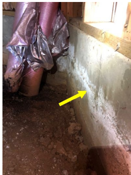
Efflorescence on foundation wall
