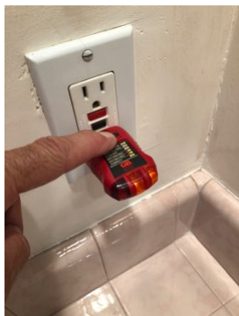
Deficient bath 2 GFCI with power on
