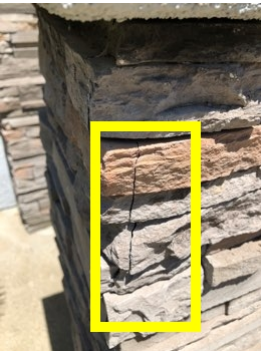
Deck railing stone column cracking
