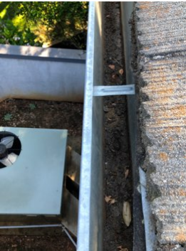
Organic material in gutter
