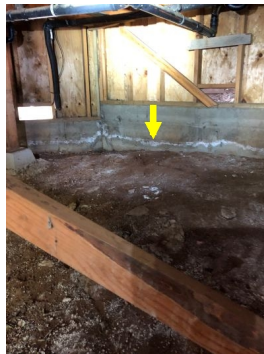
Efflorescence on foundation wall
