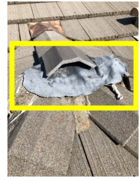
Questionable right ridge junction repair
