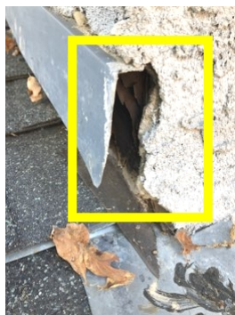
Front gap in flashing
