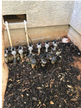
Irrigation system sprinkler valves
