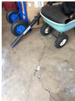
Significant concrete floor cracking
