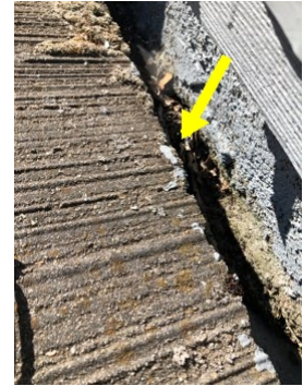
Clogged chimney 2 upper flashing
