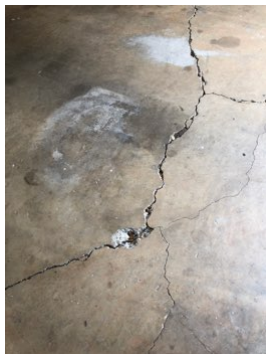
Significant concrete floor cracking
