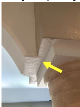
Left living room column crack
