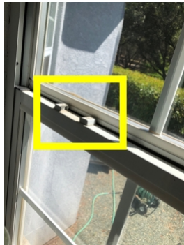
Broken latch in toilet room
