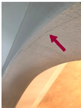
Dining archway cracking
