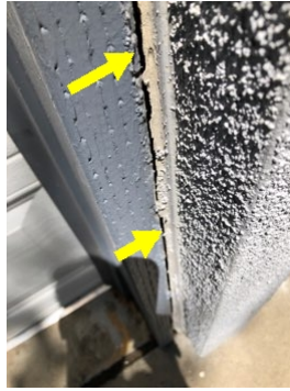
Deficient left vehicle door seal
