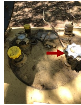
Liquid propane tank shut-off valve detail
