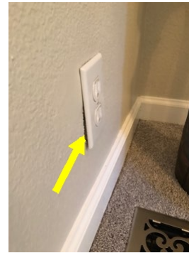
Dining room outlet not flush to wall
