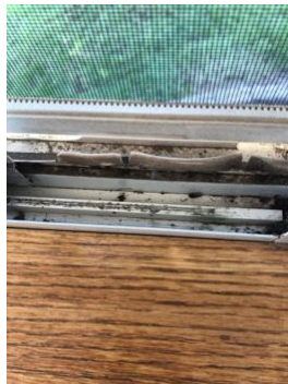
Cracked window screen seal
