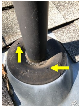
Holes in vent pipe rubber boot
