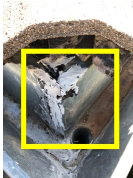
Rear right gutter seam caulk seal
