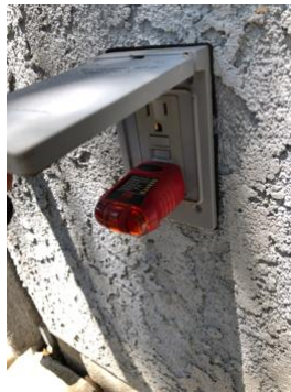
Deficient front right GFCI outlet
