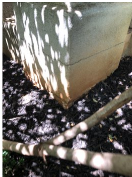
Left column bottom cracking
