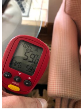
Great room cooling system register temp
