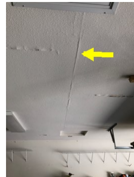
Lifting seam tape
