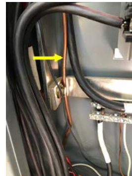
Grounding electrode wire detail
