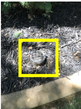
Front drain grate detail
