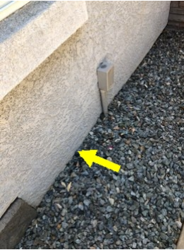
Weep screed covered on right side
