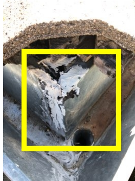
Rear right gutter seam caulk seal
