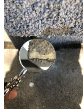
Exposed bottom foam on front trim
