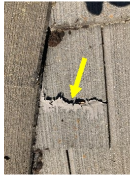
Patched right side tile
