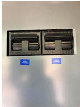
200 amp X 2 main breaker detail
