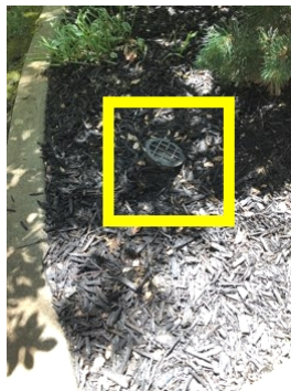
Front drain grate detail
