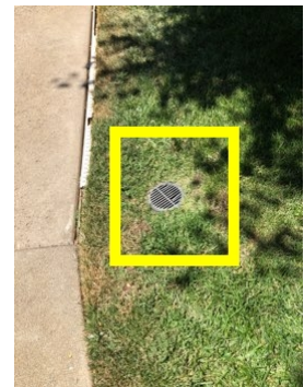
Rear drainage grate detail
