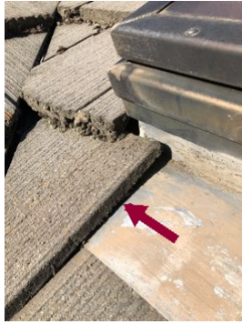
Skylight flashing under tile
